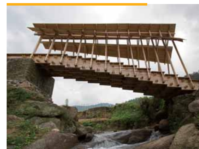
Architecture students joined hands with local craftsmen to build a timber footbridge on the Chinese Mainland, experiencing different building methods and challenges 建築學院學生在內地與當地工匠攜手搭建木橋，體驗不同的建築方法與挑戰
